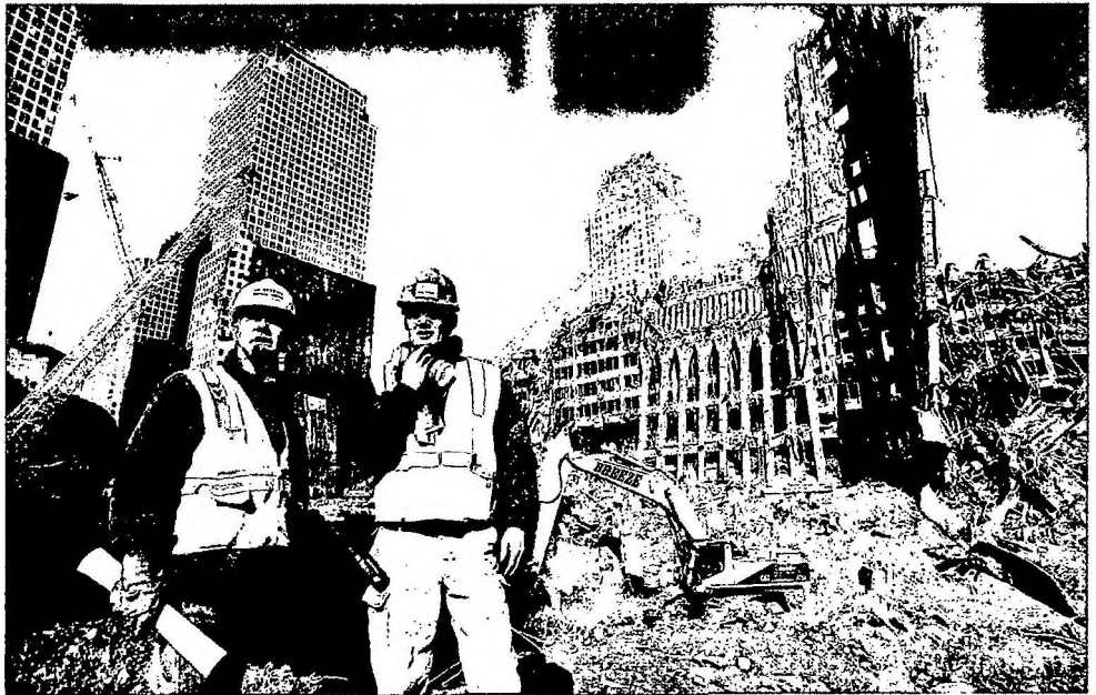
ASSESSMENT Slattery Skanska's McGuinness (left) and Koch Skanska's Matre review damage.
