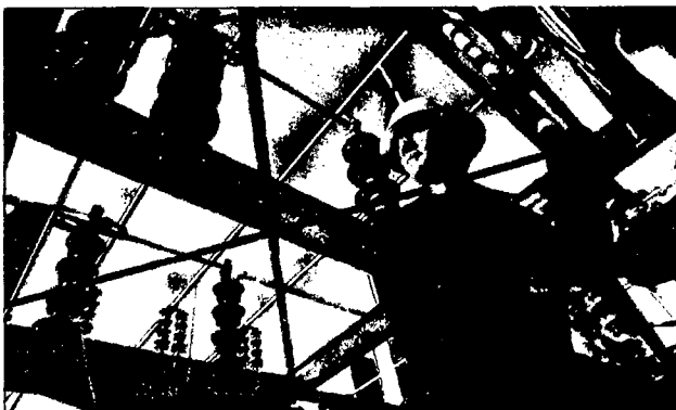
E.S. Boulos builds substations throughout the Northeast.
