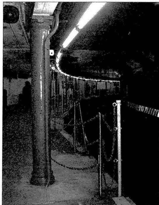
The curved, outmoded South Ferry Platform.
