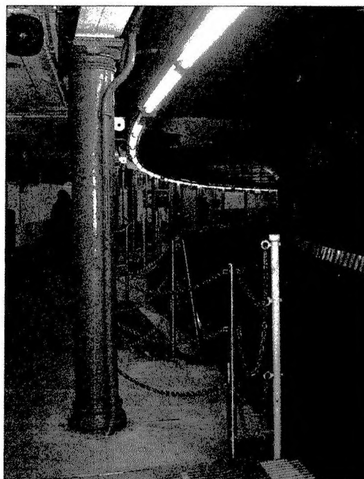
The curved, outmoded South Ferry Platform.
