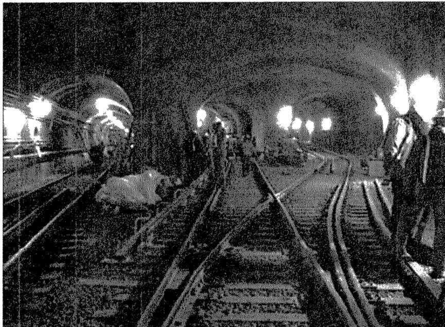
The Port Authority is creating new crossover tracks at Exchange Place in Jersey City to enable PATH service restoration at that station by June 2003.
