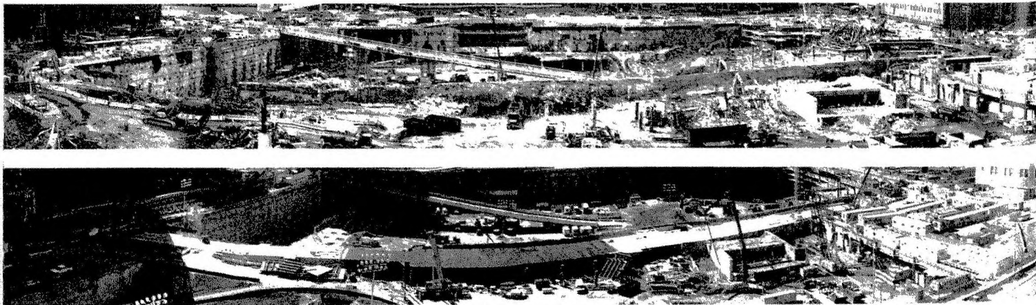
MOVING ON With clear site at Ground Zero, transit repairs ramped up last spring (top). Subway line is now visible (below).
