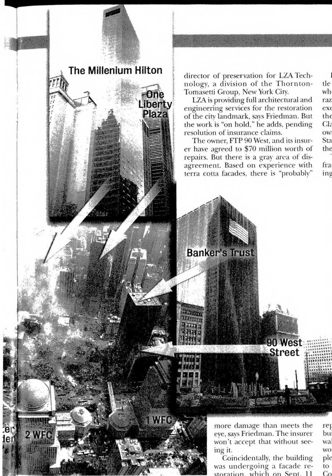
PERIPHERAL BUILDINGS Insurance issues and open questions about the area's redevelopment have stymied fixes of some, but not all, WTC neighbors.
