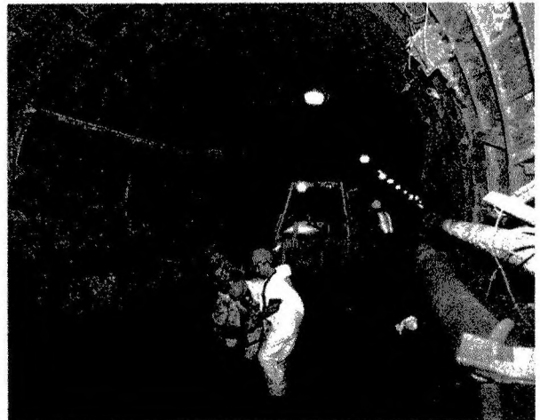
STRIPPED PATH tunnels get new conduit and track.
