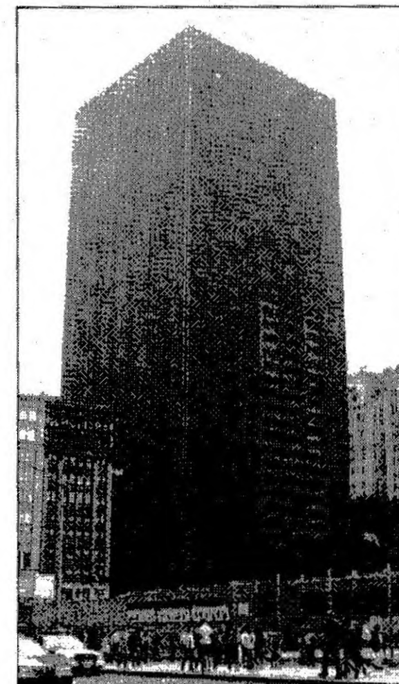
The abandoned Deutsche Bank building was severely damaged when the south tower collapsed and will be demolished in the future.
