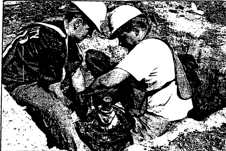
HEAVY DUTY WORK: Local 376 Construction Laborers in Dept. of Environmental Protection remove top of buried high-pressure fire hydrant, a remnant of an unused system of underground pipes that the city may now sell as conduits for fiber-optic computer communications. Their local recently emerged from administatorship, more democratic and more aggressive than before.
