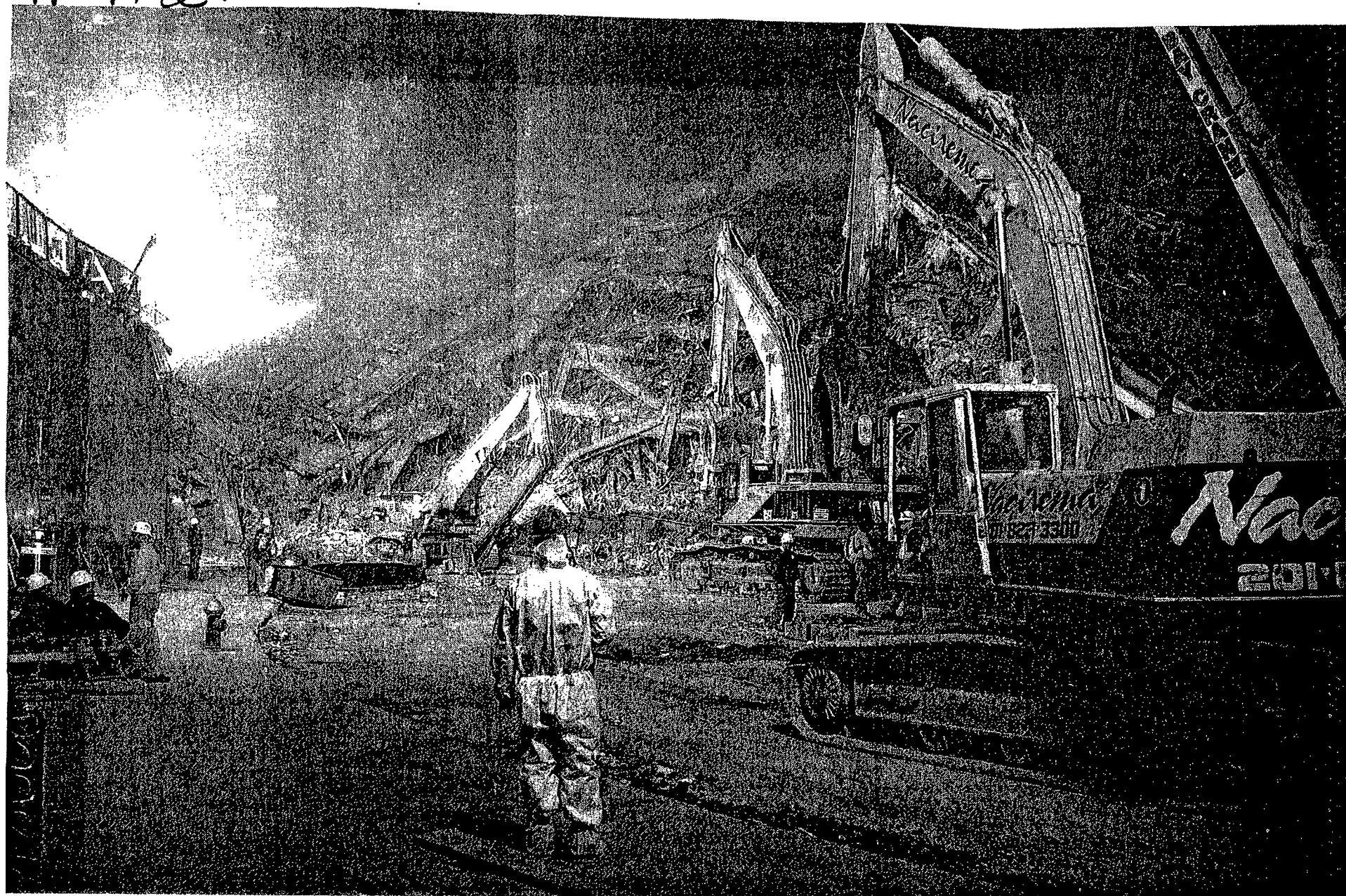
Edward Keating/The New York Times A worker stood next to heavy equipment of Nacirema Industries engaged in search and rescue yesterday at the trade center collapse site. Efforts are shifting toward demolition removal.
