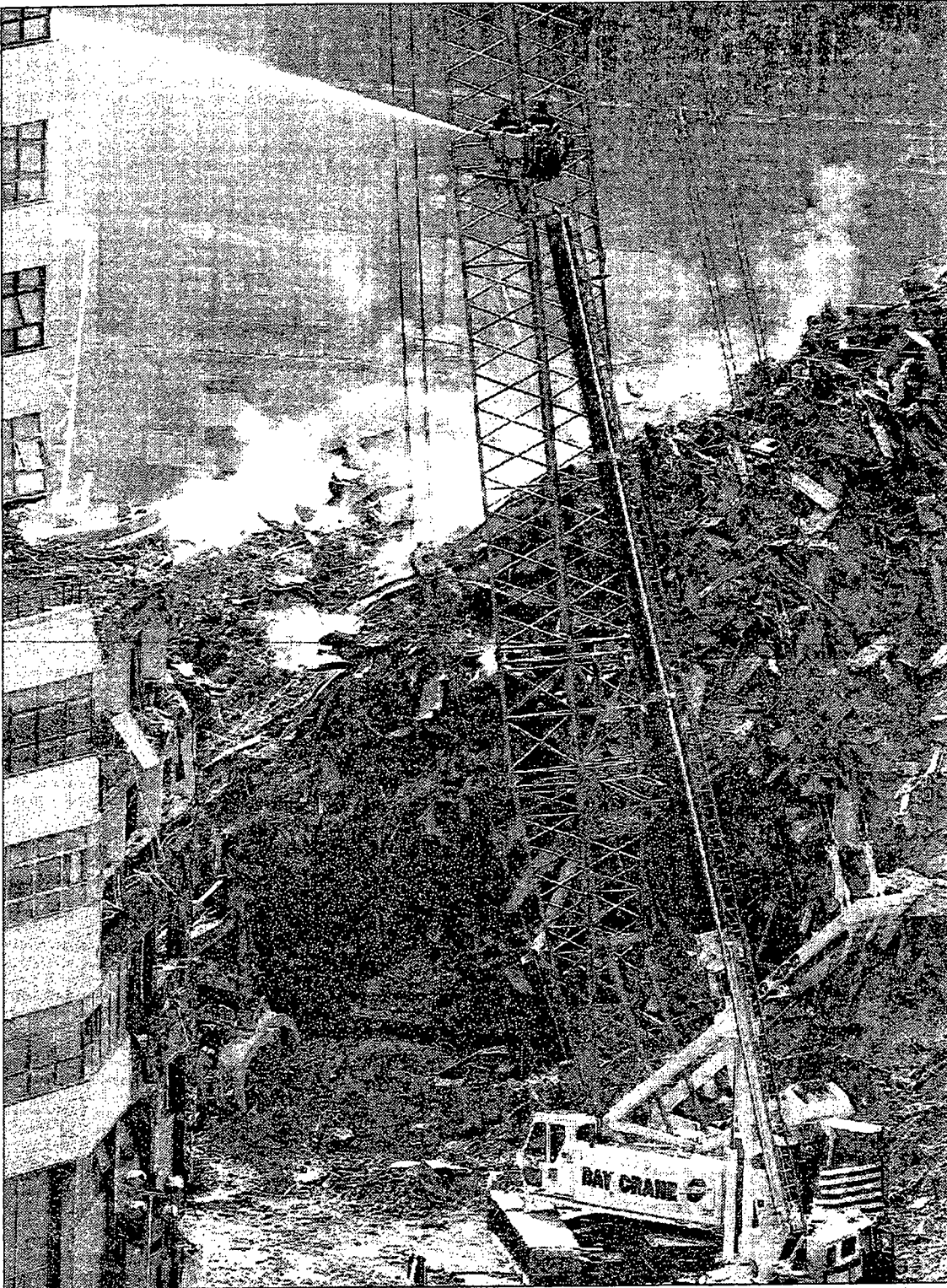
DAUNTING TASK The tough, dangerous work of removing the wreckage of the World Trade Center terrorist attacks goes on day and night, with Mayor Giuliani saying it could take a year.
